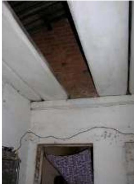
**13 HOUSE, THE EXTERIOR OF WHICH IS CRACKED AND THE INTERIOR WHICH HAS PARTIALLY FALLEN DOWN BECAUSE OF EXPLOSIONS IN THE T17 MINE IN MUSONOI**
