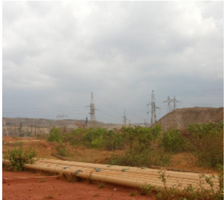
**IN THE FOREGROUND, THE WHITE PIPES TRANSPORTING THE ORE FROM THE KAMOTO CONCENTRATOR TO THE LUILU HYDROMETALLURGICAL PLANT. IN THE BACK, THE DARKER PIPES CARRYING WATER TO LUILU AND WHICH HAVE BEEN PUNCTURED AND STOLEN.**
