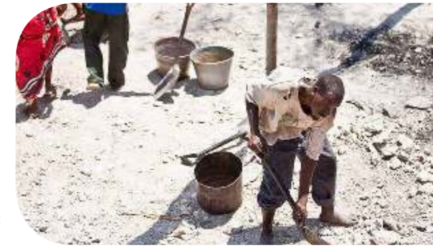
Building a reservoir in the Central Region.
