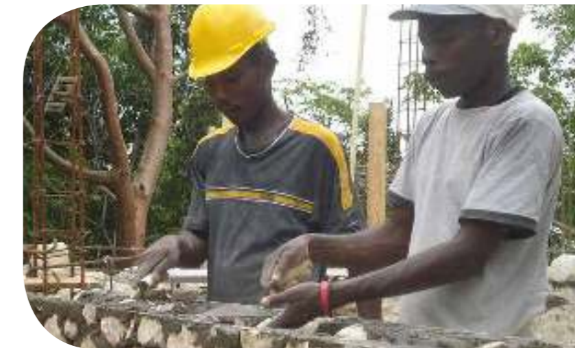
Construction work in Artibonite.
