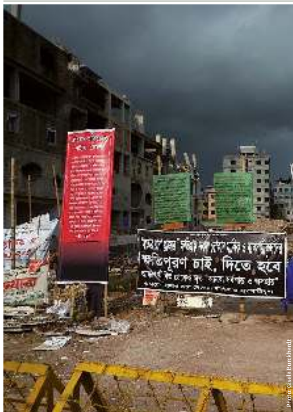
The collapse of the Rana Plaza building in Bangladesh caused over 1100 deaths.
